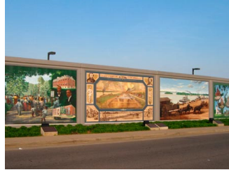
Padukah, Kentucky Floodwall, 2007
