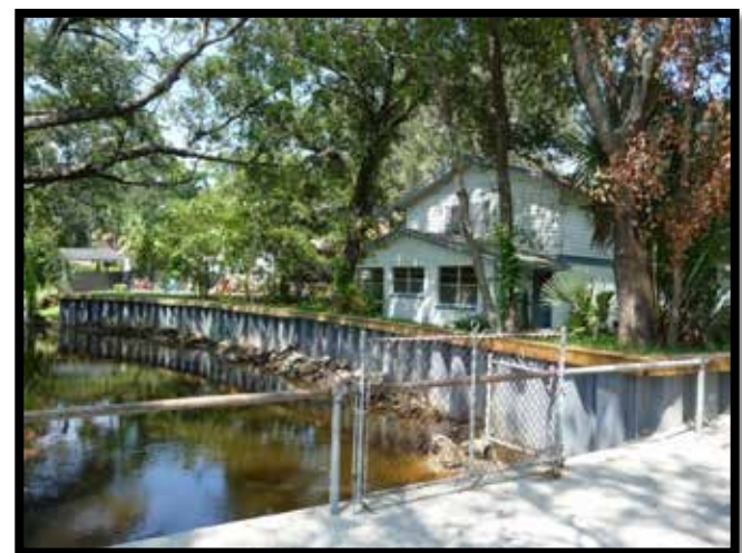
Post-mitigation image of project site for FMA-PJ-04-FL-2008-001 (photo courtesy of City of Jacksonville).
