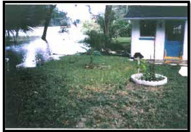
Pre-mitigation image of project site for FMA-PJ-04-FL-2008-001 (photo courtesy of State of Florida).
