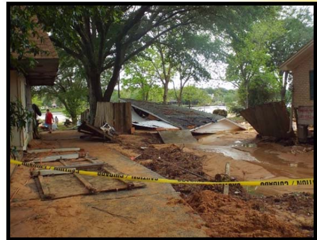
Flood damage in Pensacola, FL. Source: Pensacola News Journal
