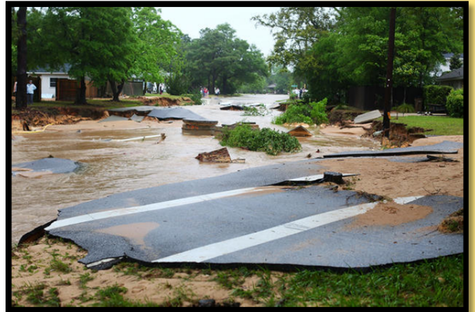
The road bed of Piedmont Street crumbles after it washed out due to heavy rains. Source: Getty Images, Marianna Massey
