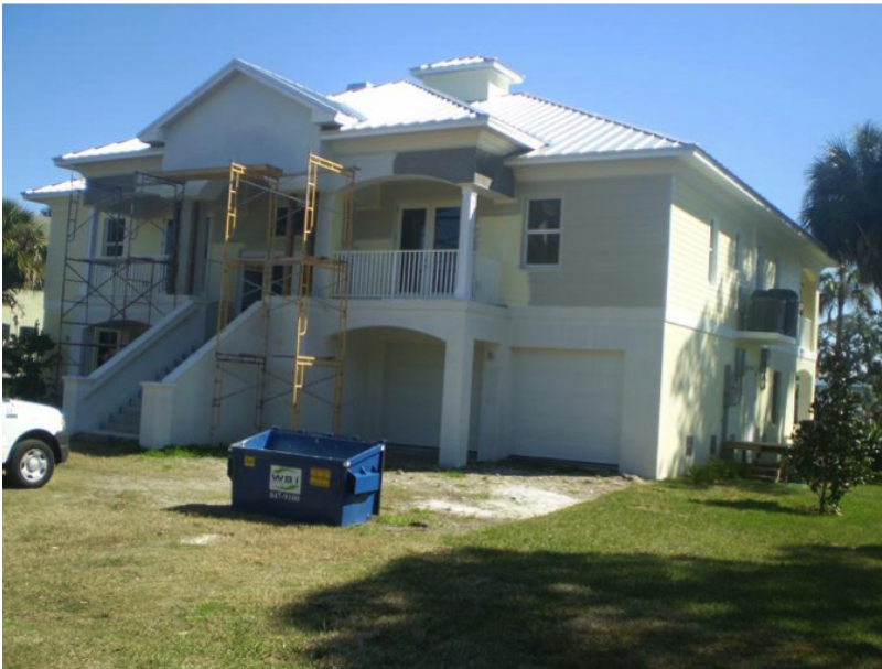
Figure 7: Pasco County Reconstruction Site Structure During Mitigation
