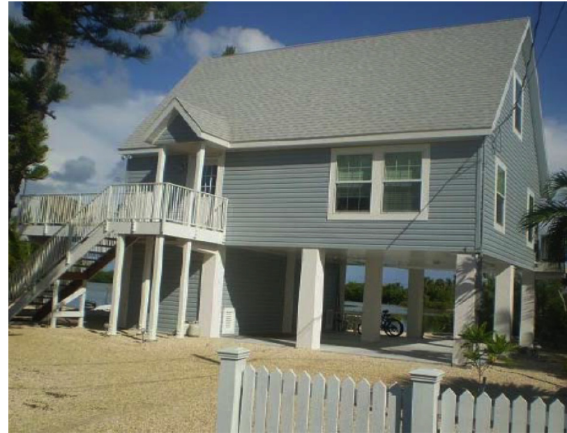
Figure 5: Monroe County Reconstruction Site Structure After Mitigation
