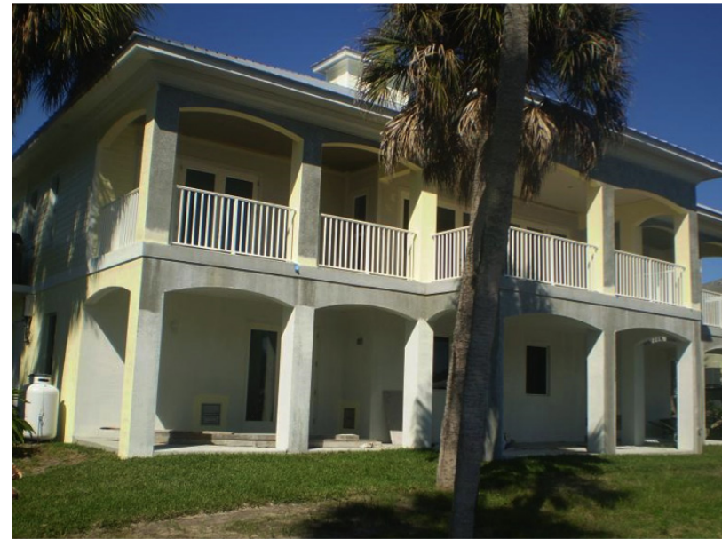
Figure 8: Pasco County Reconstruction Site Structure After Mitigation
