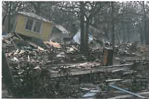
Without mitigation techniques applied, your home may not withstand a windstorm as well as you think it will.
