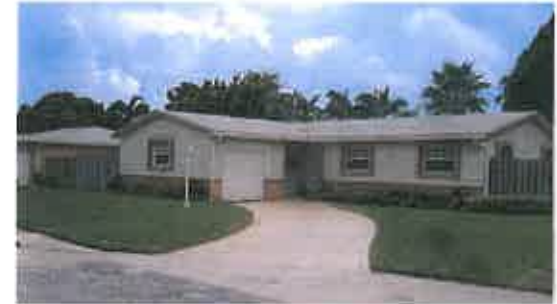
This home is classified as "gable roof".
