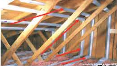
These are examples of "gable end reinforcements".
