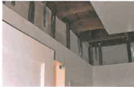
Photo above shows roof to wall connections.
