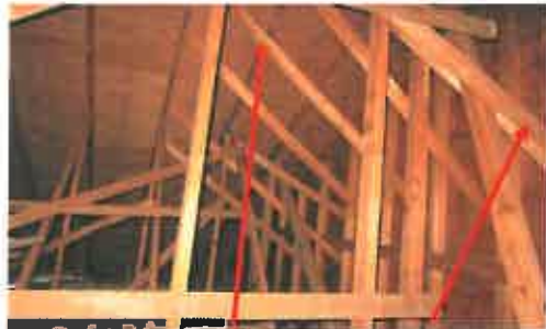
These are examples of "gable end reinforcements".
