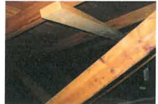
This photo shows a form of bracing.
