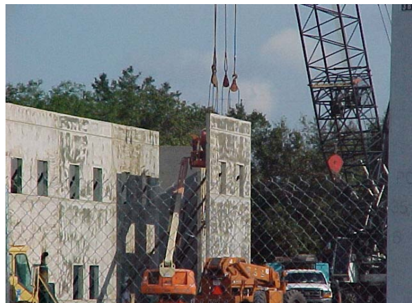
Figure 4-2. New school facility being constructed to the public shelter design criteria.
