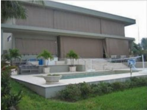
Outside and inside views: A screen protection system enclosing an entire porch or lanai helps to keep wind and flying debris away from the openings. As a result, you may opt to leave your patio furniture or other loose items from your yard outside for minimal hurricanes which saves on preparation time. For strong or severe hurricanes you may want to bring all loose items into the house or garage. Note the custom fit on the decorative column caps.
