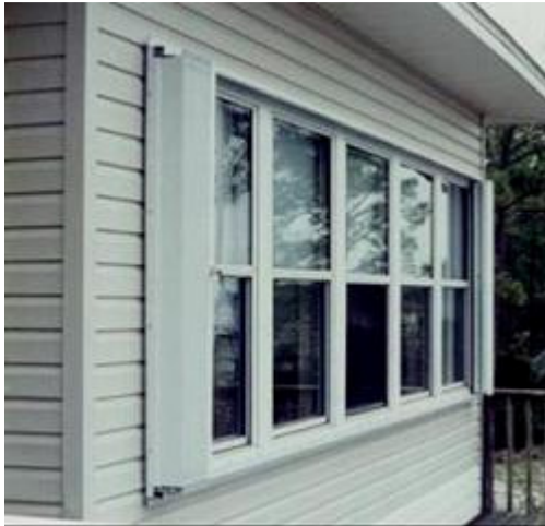
Typical images of stored and activated accordion shutter system
