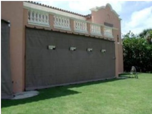
Outside and inside views: A screen protection system enclosing an entire porch or lanai helps to keep wind and flying debris away from the openings. As a result, you may opt to leave your patio furniture or other loose items from your yard outside for minimal hurricanes which saves on preparation time. For strong or severe hurricanes you may want to bring all loose items into the house or garage. Note the custom fit on the decorative column caps.
