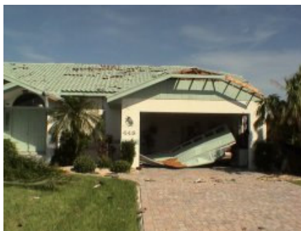
Garage door blown in on top of car
