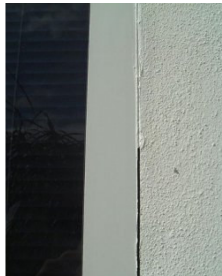
A long gouge next to a window to be Partially sealed gouge sealed with urethane caulk
