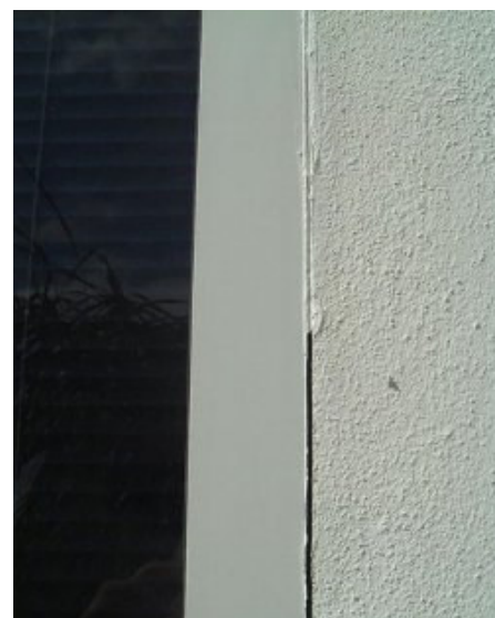
Partially filled gap
