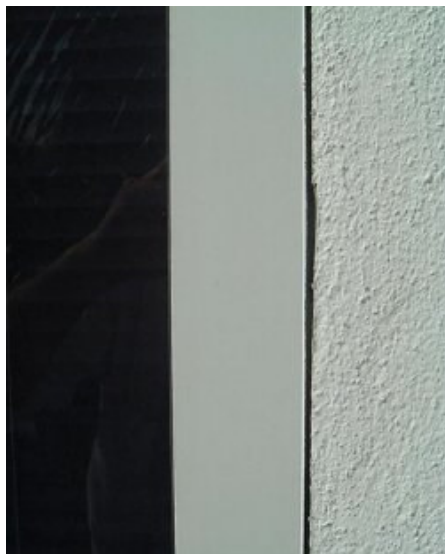
A long gouge next to a window to be Partially sealed gouge sealed with urethane caulk
