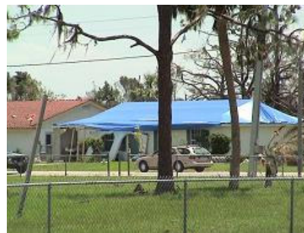
Temporary protection after storm damage to roof
