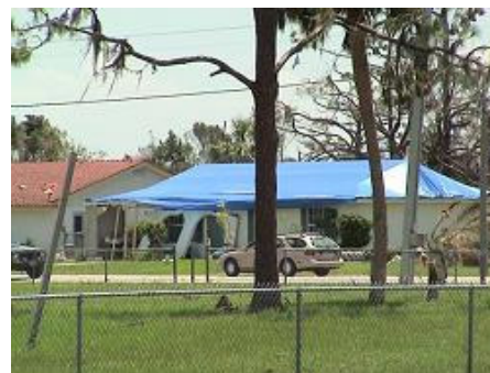
Temporary protection after storm damage to roof
