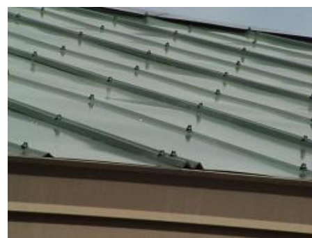
5-V crimp metal roof with external fasteners - makes it easy to see how well the metal is anchored to the roof deck (click image for larger version)
