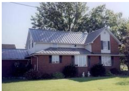
Standing metal seam roof (click image for larger version)
