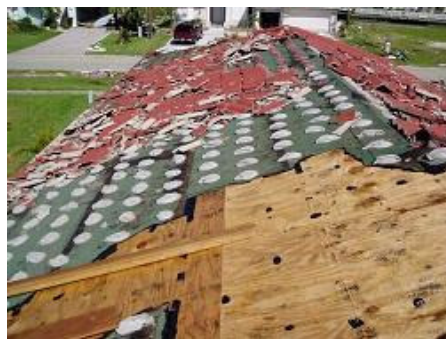
Mortar set files rely on adhesion of file to mortar and mortar to underlayment
