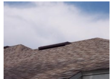
Off-ridge vent on a shingle roof
