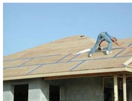
Installing secondary water protection over seams between roof sheathing
