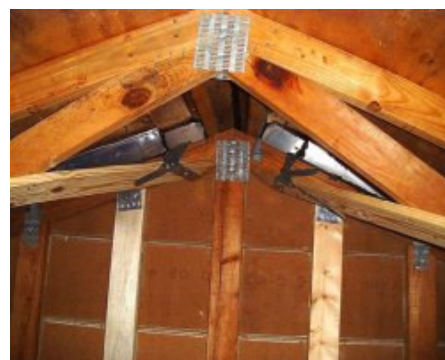
Sketch of gable roof structure with Note aluminum flashing installed and outrigger system showing water entry caulked to block water entry during point through gable soffit vent hurricane
