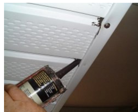
Screw installed through wall J channel and through soffit panel and hopefully into wood above - black caulk shown for contrast. You can usually find screws that also match trim color.
