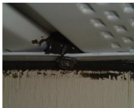
Screw installed through wall J channel and through soffit panel and hopefully into wood above - black caulk shown for contrast. You can usually find screws that also match trim color.
