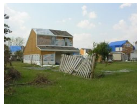
House missing its vinyl siding (click image for larger version)
