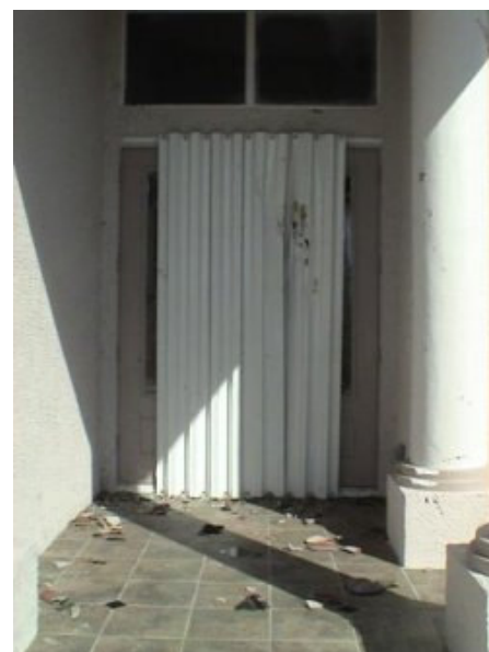
Shuttered entry door
