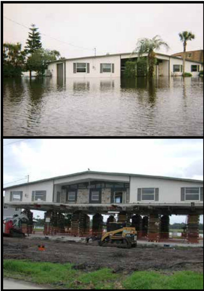
Structure flooded by Tropical Storm Fay and mitigation of the same structure in progress (photos courtesy of Volusia County)
