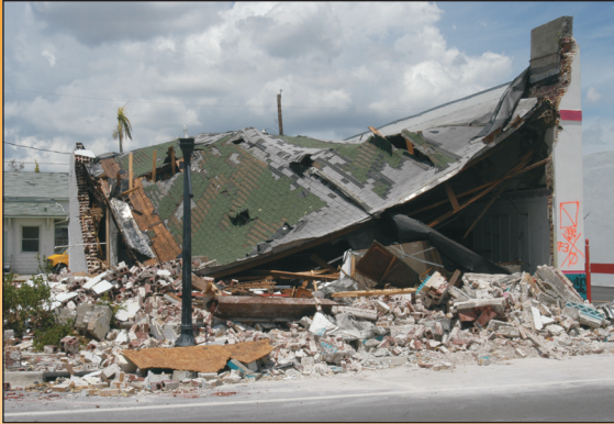
Collapsed structure requiring replacement
