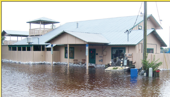
Flood control measures such as sandbagging could be an eligible Category B project
