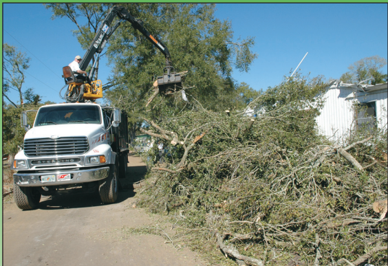
Vegetative debris removal
