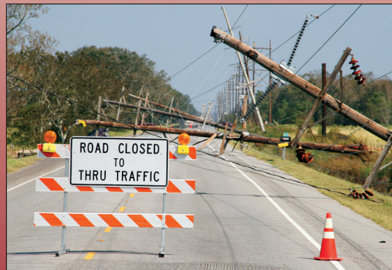
Downed utility poles blocking a road
