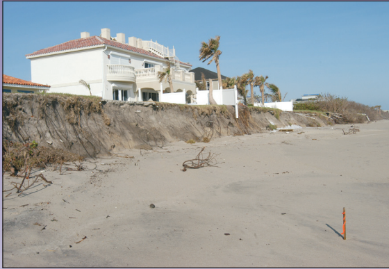
Beach erosion caused by high seas
