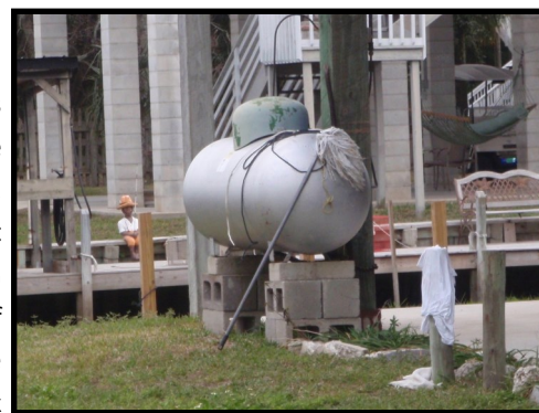
Picture above is an unanchored tank.
