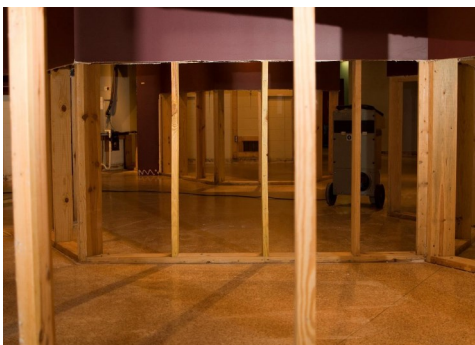
Above: Large fans were used to dry out the water-damaged West Wing of the Daytona Beach Museum of Arts & Sciences (MOAS) after the devastating flood of 2009. Photo courtesy MOAS.
