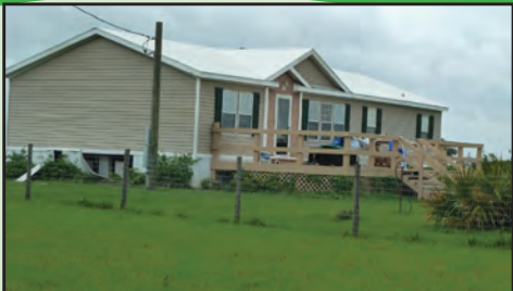
Affected Manufactured Home, skirting affected
