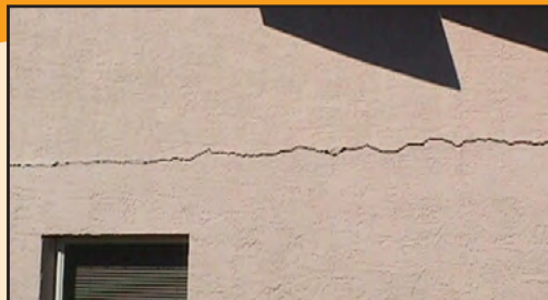
Structural cracks—roof lifted, Single Family (SF)
