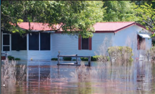
Minor: 10," standing water, Single Family (SF)
