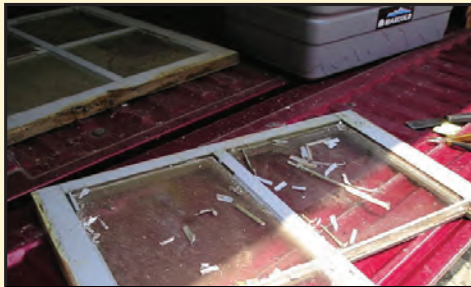
Window frames broken
