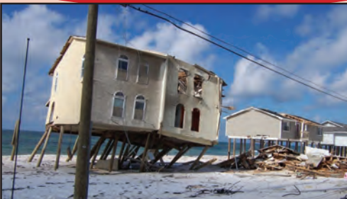
Foundation, roof, walls unsound, Multi-Family (MF)
