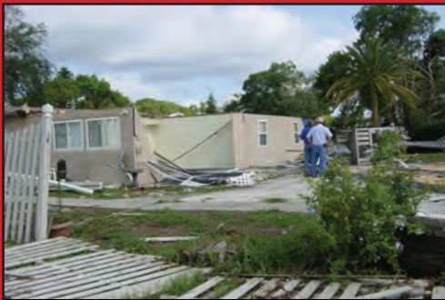
Roof & walls collapsed, Single Family (SF)
