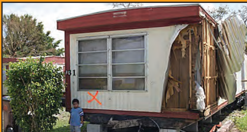
Wall coverings damaged and exposed, Manufactured Home (MH)
