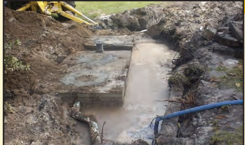
Flood septic tank damage
