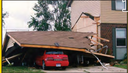
Damage to wall small breach, Multi-Family (MF)
