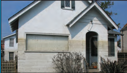
Destroyed: 5,' standing water, Single Family (SF)
