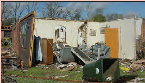
Roof gone, walls collapsed, Manufactured Home (MH)
