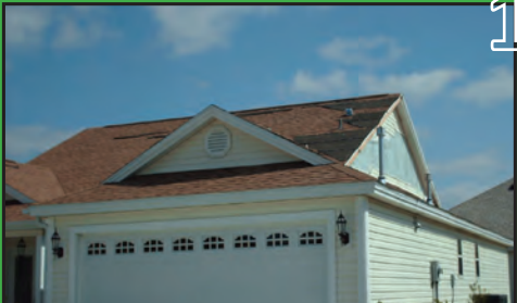
Few missing shingles, covered, no impending weather
