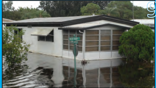
Major: 3," standing water, Manufactured Home (MH)
