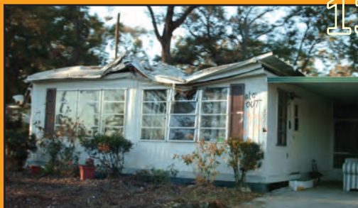
Roof partially collapsed, Manufactured Home (MH)
