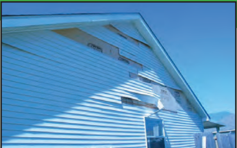
Loose and missing siding
