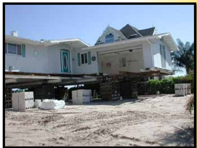
The average cost per structure elevated was about $265,000 for projects included in this assessment (photo courtesy of Volusia County, Florida)
