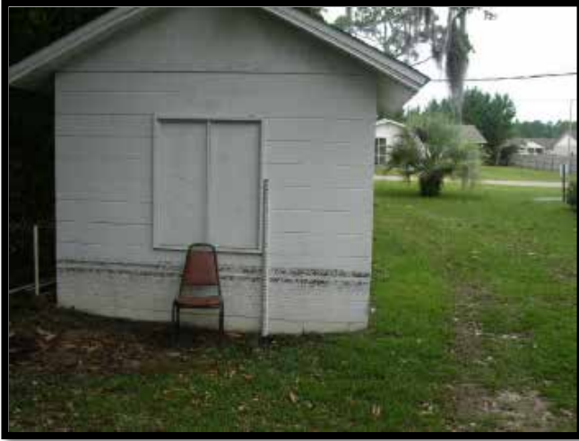
High water marks were collected and generously provided by some of Florida's Water Management Districts (photo courtesy of the Northwest Florida Water Management District)
