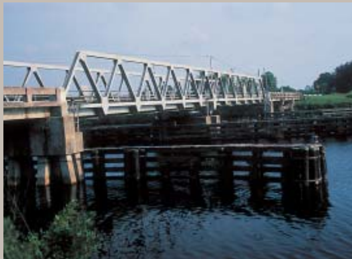
STRUCTURE—Ft. Denaud Swing Bridge, Hendry County. FLORIDA DEPARTMENT OF STATE
