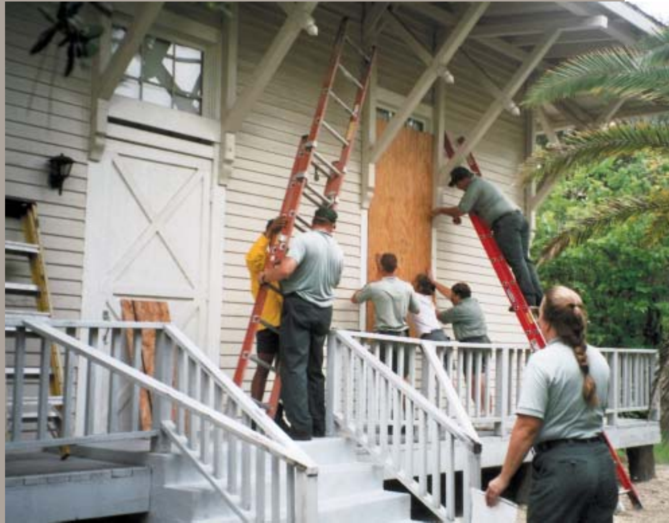
The Art Hall at the Koreshan State Historic Site is "battened down" for a storm. KORESHAN STATE HISTORIC SITE
