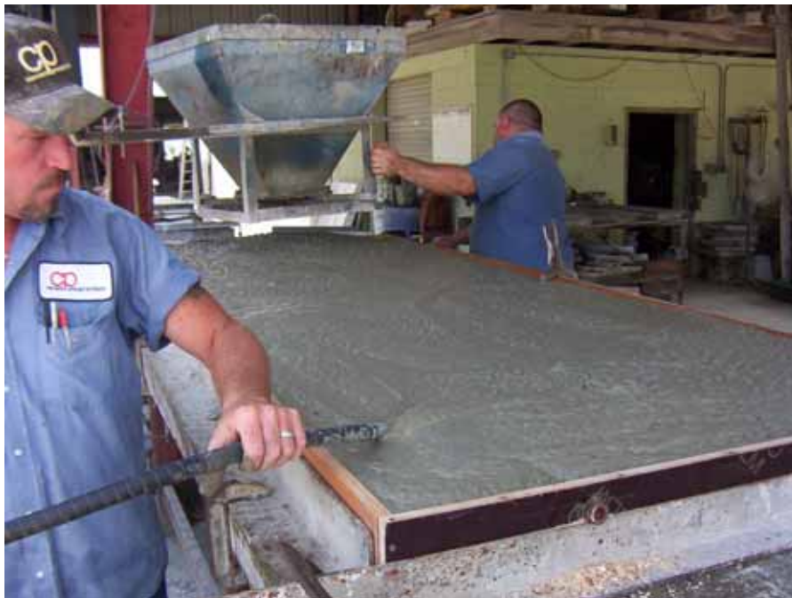
Figure 3.17: Construction of the Tilt-up Panel
