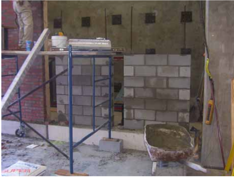
Figure 3.18: Construction of CMU Specimen
