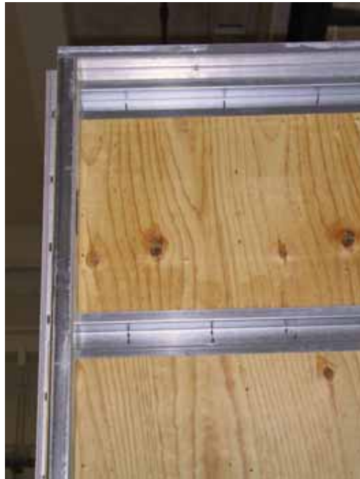
Figure 3.21: Plywood Attached to Purlins
