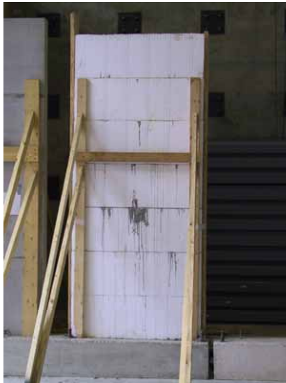
Figure 3.19: Completed ICF Specimen
